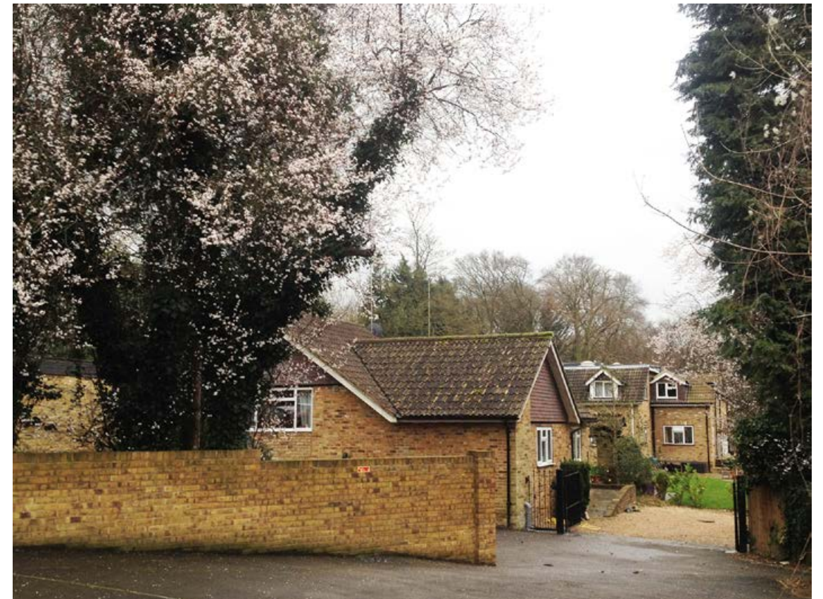
Elderly People's Home back-land 2-storey development with dormer roofs
