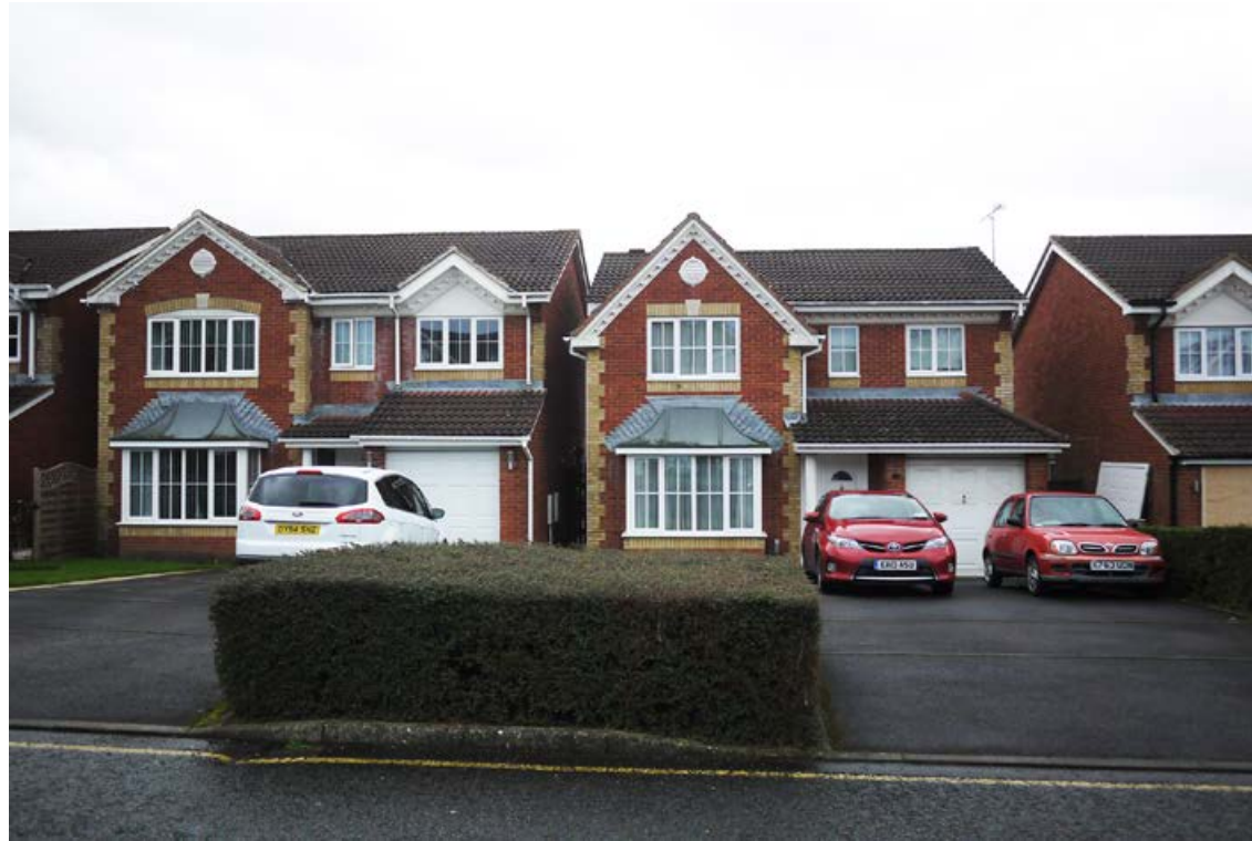
Consistent approaches to facade treatment and proportions create a uniform townscape
