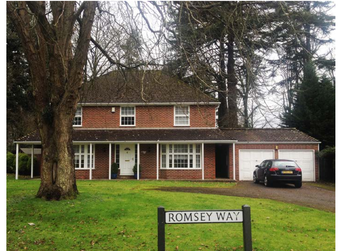
Example of 2-storey porched villa with integrated garage and surrounded by mature trees
