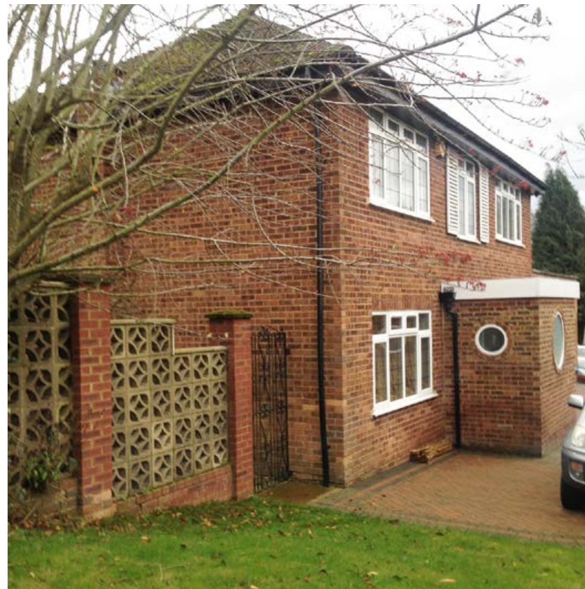
Decorative brick wall and extended entrance volume
