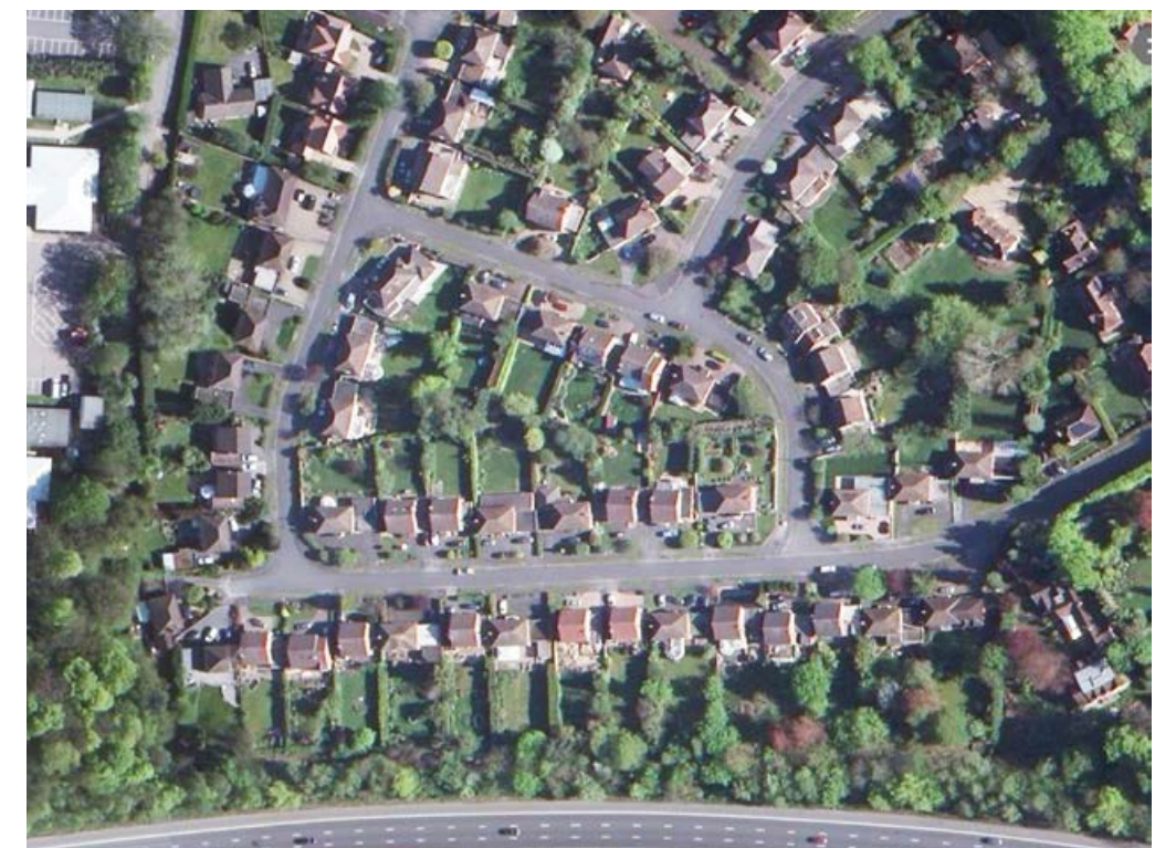
Character Zone C Aerial view ( Google maps )
