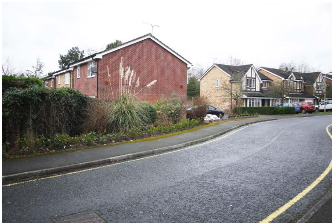
Typical street width and soft-edge boundary treatment
