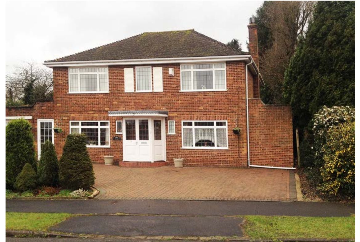
2 storey red brick villa with central protruding entrance and paved front garden
