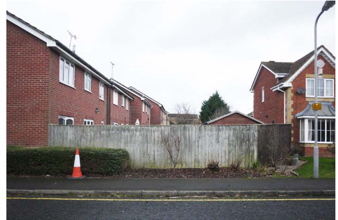
Timber-fence boundary treatment creates an unsatisfactory edge to the street
