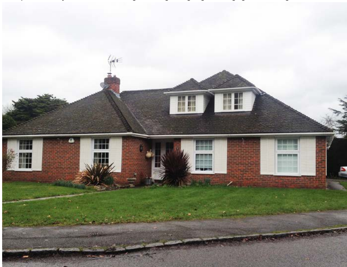
Example of 1-storey suburban villa with dormer extensions
